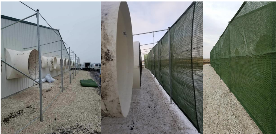
Figure 1. Installed electrostatic precipitator and geotextile fence system.
